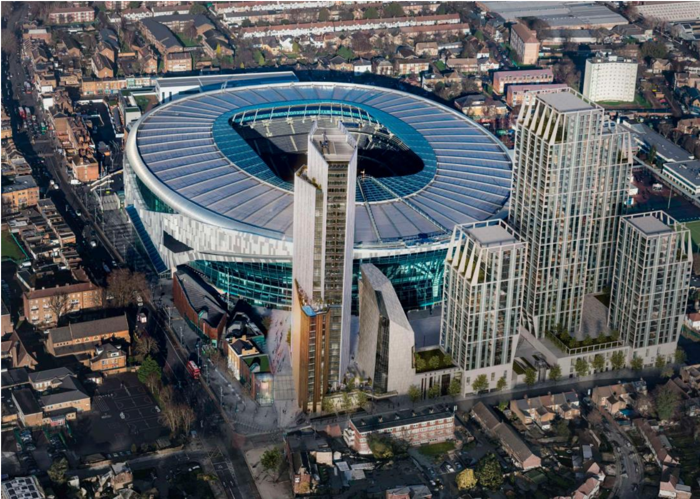
OVERVIEW AERIAL IMAGE FROM SOUTH OF HIGH ROAD
